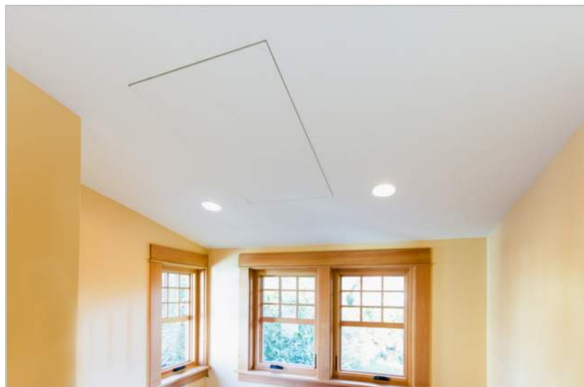
Figure M4: Radiant Ceiling Panel Option
