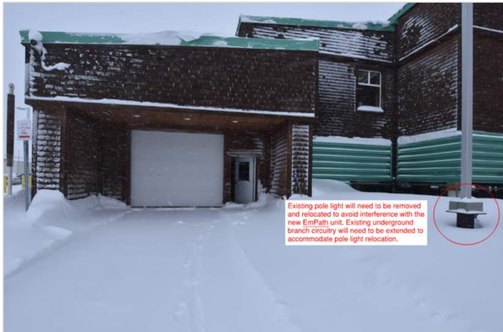
Figure E3: Existing Exterior Light Pole
