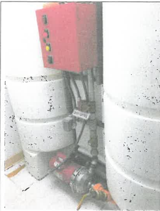
Photo M1 – Sprinkler Storage Tank
