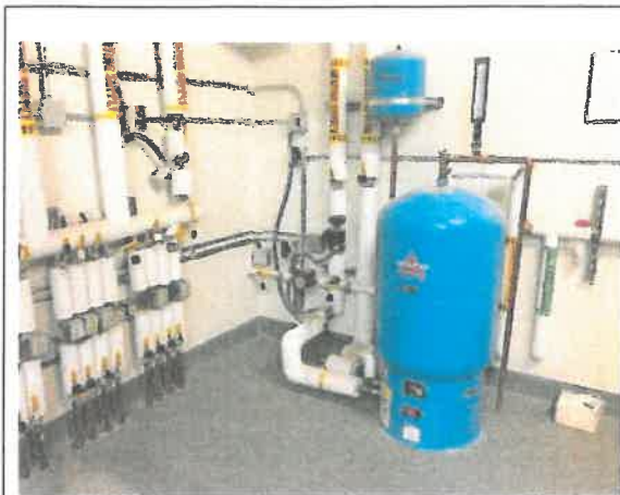
Photo M5 – Hot Water Generator
