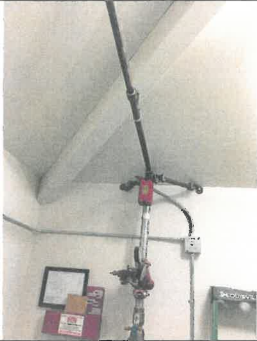
Photo M1 –Sprinkler Valve
