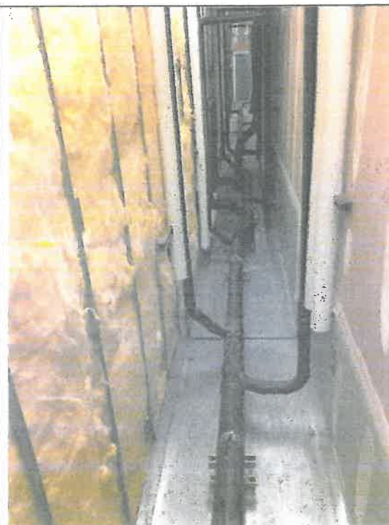
Photo M2 – Waste Piping in Chase
