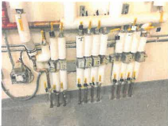
Photo 9 – Fin-tube Control Valves
