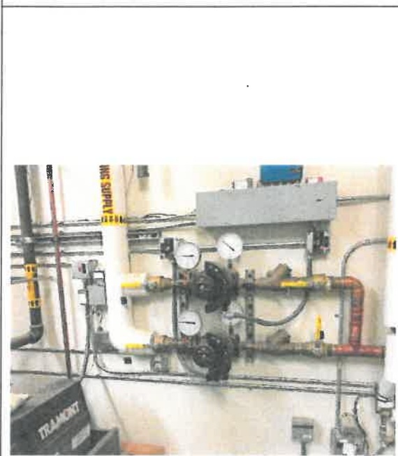
Photo M7 – VFD Heating Pumps
