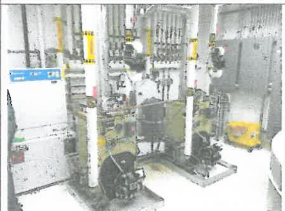
Photo M5 – Hot Water Generator
