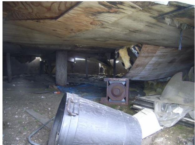
Collapsed floor shown underneath
