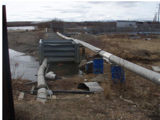
Waste water discharge to lagoon (top pipe), City water source line from river (lower pipe) to water treatment plant
